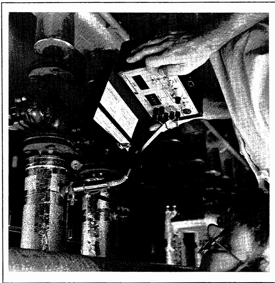
Fig. 8/4: Monitoring of pressure in pipes (Photo: Hottinger Baldwin Messtechnik GmbH)
